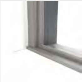
↑ Threshold only 30 mm in height.
